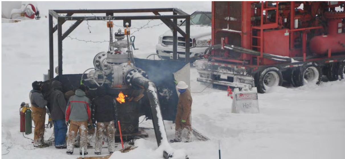
Figure 3-17. Defrosting the frozen flow line valve.
