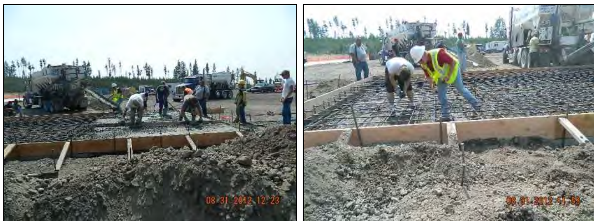
Figure 2-16. Concrete pad for stimulation pump anchor construction.
