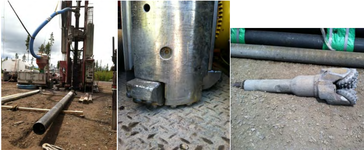
Figure 2-2. Left: advancement of casing while drilling; Center: under reaming air hammer bit with wings extended; Right: tricone drill bit used for wet borehole intervals.
