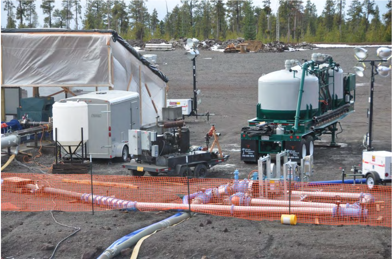
Figure 2-35. ThermoSource batch mixing unit tied into TZIM booster pump. Tracer injection set-up shown to the left of TZIM booster pump.
