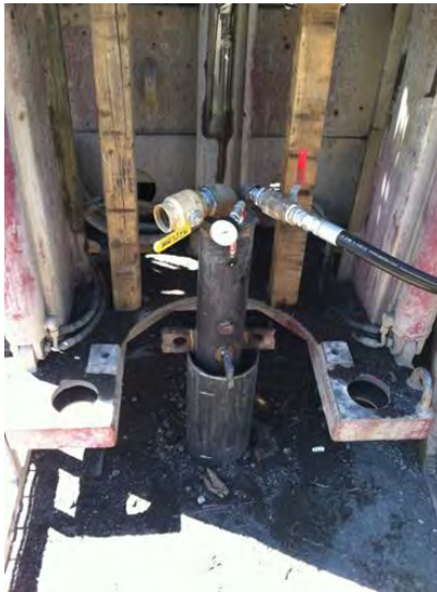
Figure 2-2. Left: advancement of casing while drilling; Center: under reaming air hammer bit with wings extended; Right: tricone drill bit used for wet borehole intervals.
